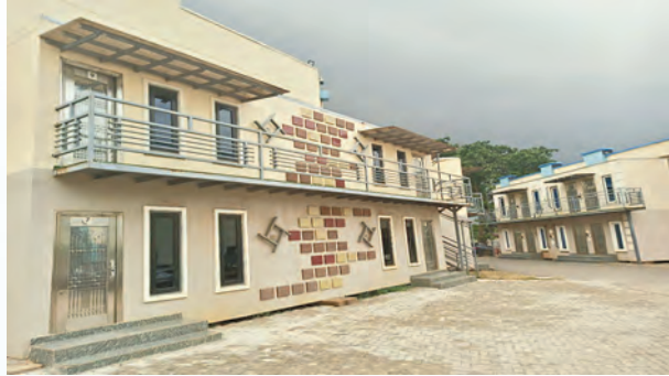
Newly installed Portacabins
