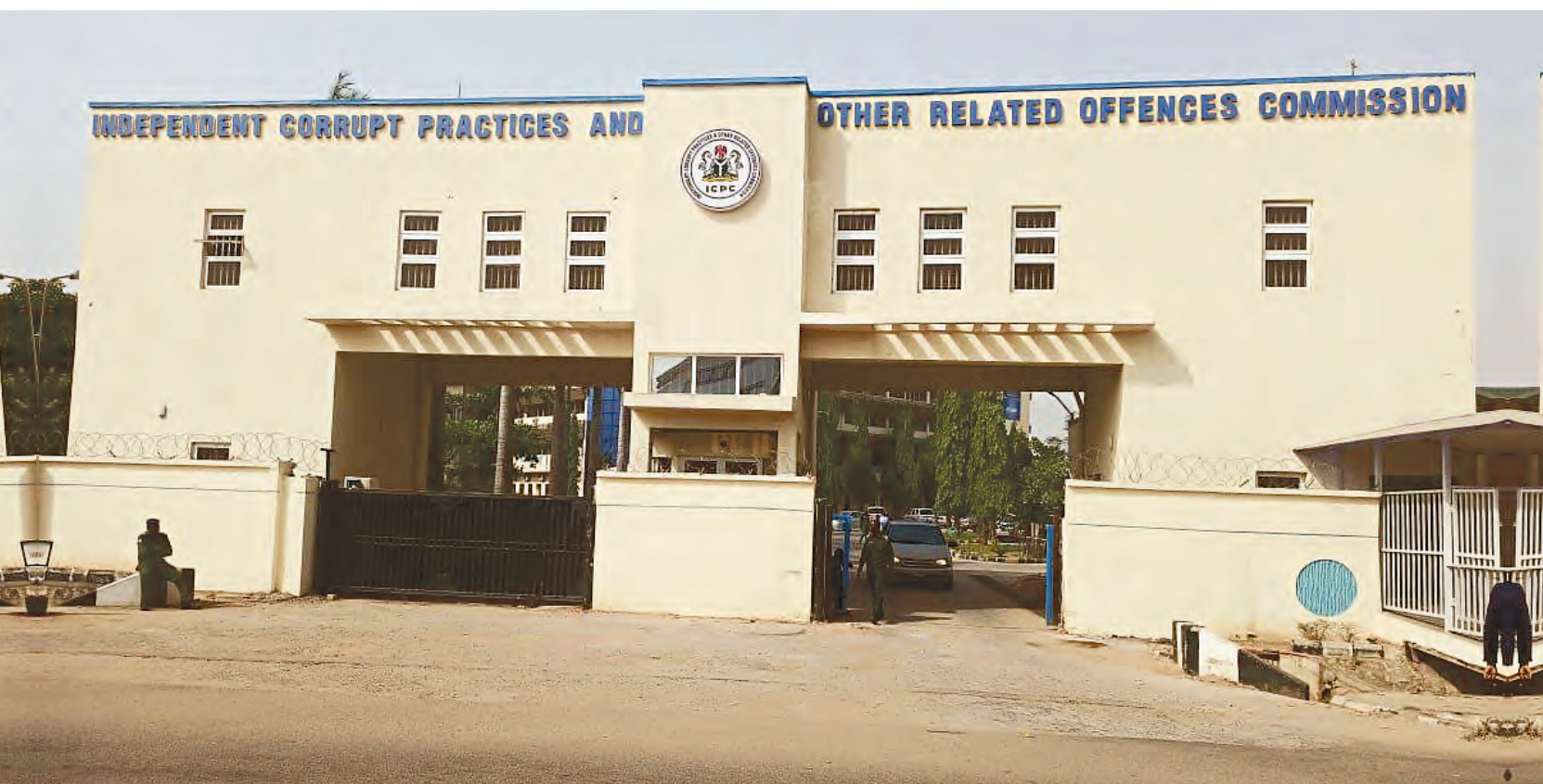
Newly Constructed Gatehouse
